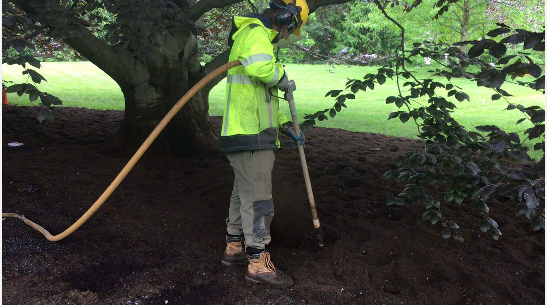
PPE for Air Tool Use: Long Sleeves, Ear Plugs and Muffs, Safety Glasses and Polycarbonate Face Shield, N95 Dust Mask or Respirator, Hardhat, Gloves, Boots
