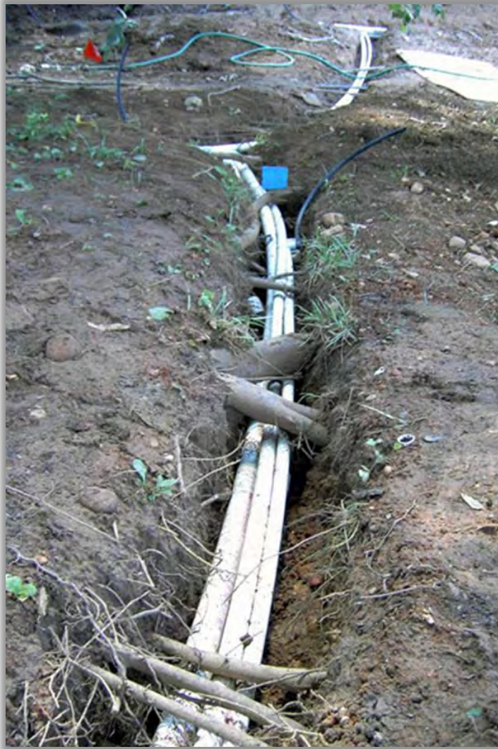
Running conduit and irrigation lines under existing roots.
