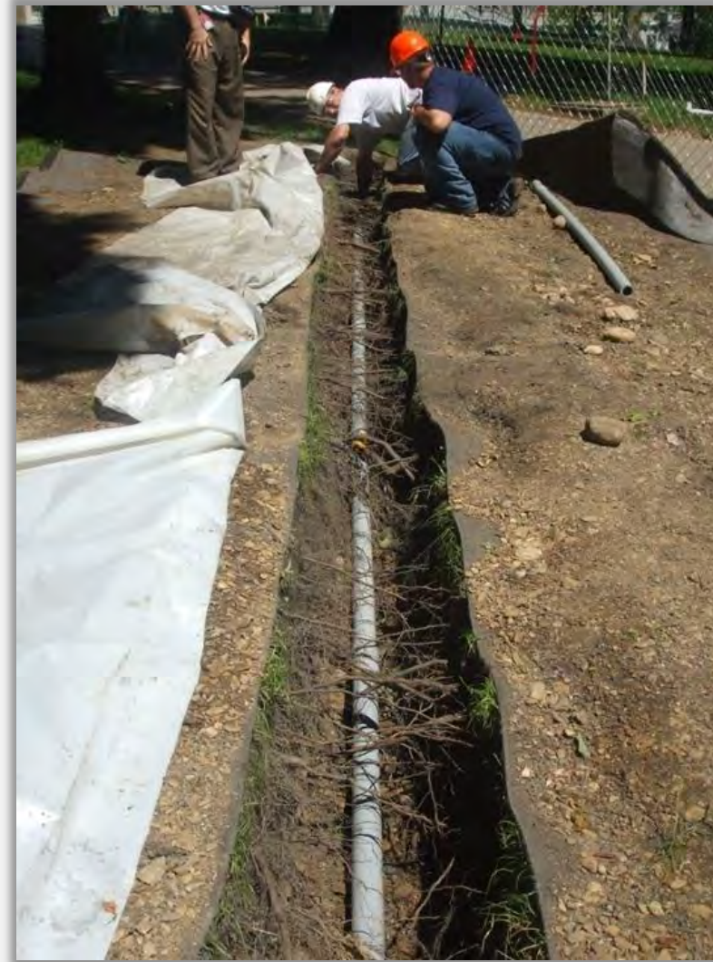
Running conduit and irrigation lines under existing roots.
